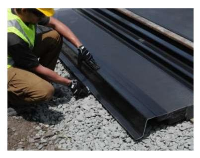
1. The *beginning* Side Track Pan should be installed with the undrilled, contoured portion of the pan at the *starting end* of the Track pan System.
