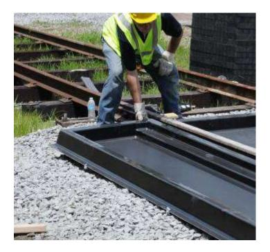
2. Loosen the bolt on two Side Pan Rail clip as far as possible without completely removing it. This will give maximum flexibility during installation of the Side Pans. You will need to use two Side Pan Rail clips for each Side Pan.
