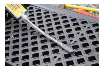
9. If using grates as a walking surface for the Railroad Track Pans, Composite Model, prepare ten grates for each Center Pan by inserting two Grating Pedestals into the diamond on the underside of each grate. These pedestals will prevent the grates from sagging over time.
