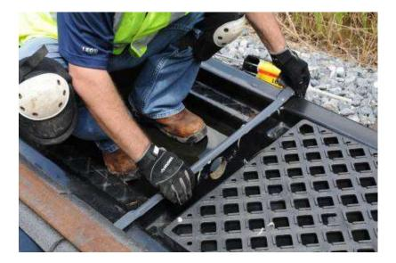
16. If using grates as a walking surface for the Railroad Track Pans, Composite Model, positon five grates in each Side Pan, using the grating locator positions on the pans.
