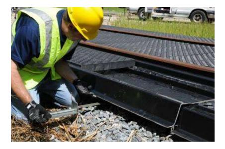
5. Stand the contoured, field-side of the Side Pan into the notches on the two "L" portions of the Side Pan Rail Clips. These "L"s will support the outside grating structure of the Side Pan and help prevent sagging and cracking over time on the field side of the Side Pan.
