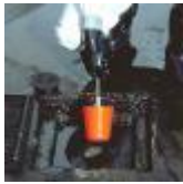
Floor Drain Plugs
