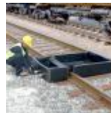
Railroad Track Berms
