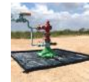
Wellhead Containment Berm
