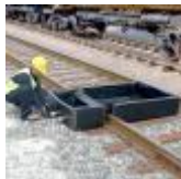
Railroad Track Berms
