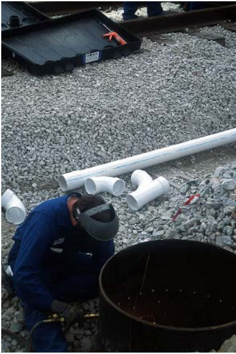
Connect pipes to sump
