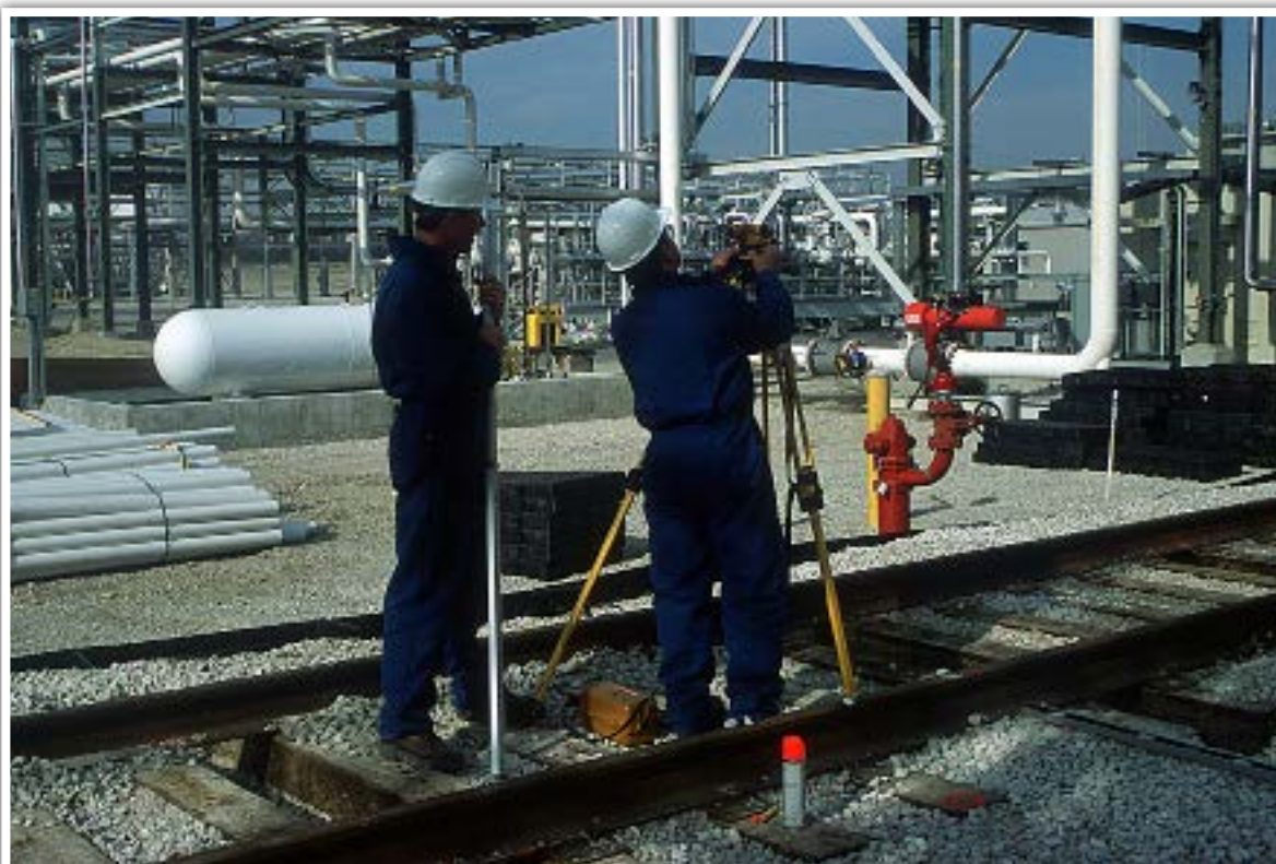
Survey to design correct slope for piping
