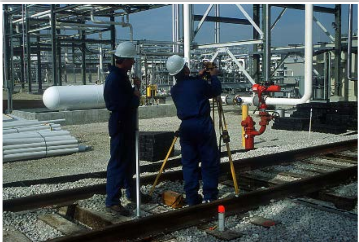
Survey to design correct slope for piping
